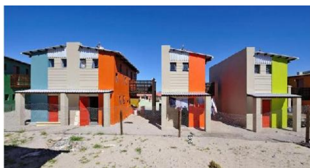
Figure 6: The duplex and single houses with in between space can be used according to individual needs (picture from presentation by Luyanda Mpahlwa, with kind permission)
