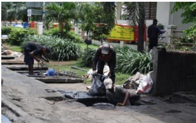
Figure 3 Local hired worker cleaning sewerage
